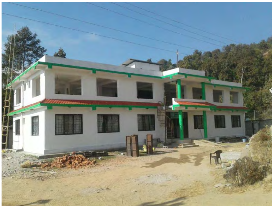
foto 9: De buitenkant is gereed (December 2016)
